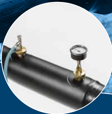
Pressure testing for leaks prior to foaming
